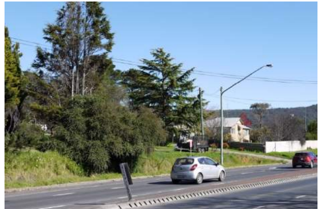
Figure 4.38 | View SW from Ironstone Cottage to No. 186 Old Hume Highway which backs onto the study site (No. 5).
