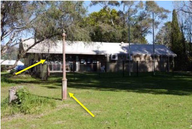
Figure 4.18 | View SW at the rear of the Cultural Centre. Highly significant are the cast iron lamp posts which were manufactured using locally produced iron at Brazenall's Foundry at Mittagong.
